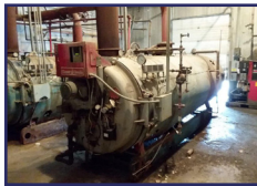
CLEAVER-BROOKS CRH263-100 PACKAGE BOILER
