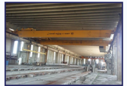
ANCHOR CRANE & HOIST 40 TON BRIDGE CRANE
