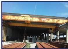
30 TON TOP RUNNING BRIDGE CRANE
